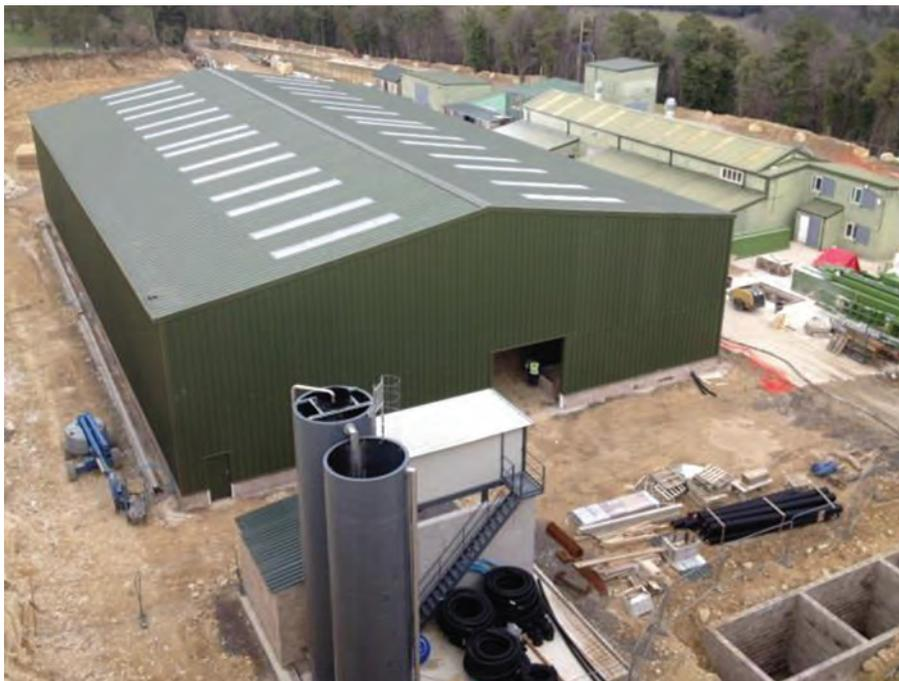
Meister Masonry's new factory in Painswick, Gloucestershire, with its OMEC water recycling system supplied by New Stone Age that will deliver 1,600 L/min of clean water.
